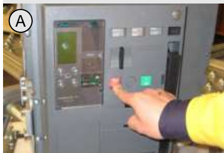
Fig. C: Device locked out
